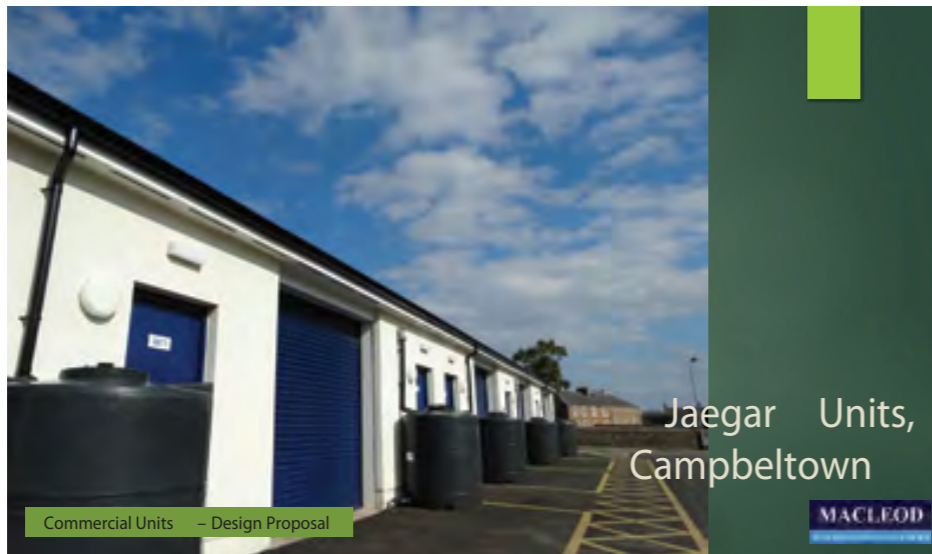
MacLeod Construction workshops at Campbeltown
