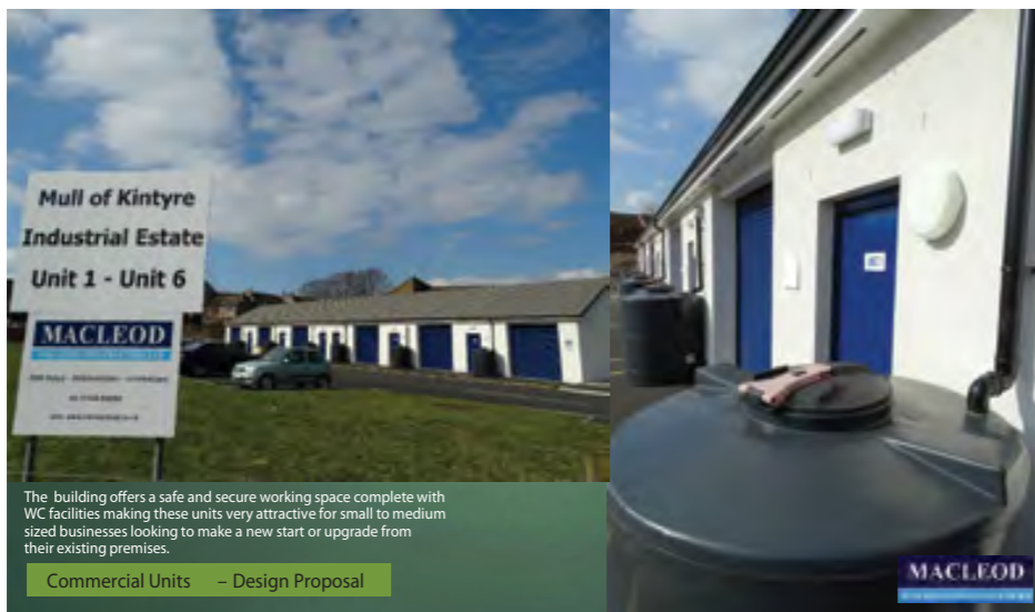
MacLeod Construction workshops at Campbeltown
